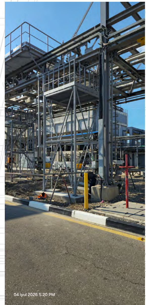
SOCAR Polymer: Installation of steam line meter platform (metal construction work)
