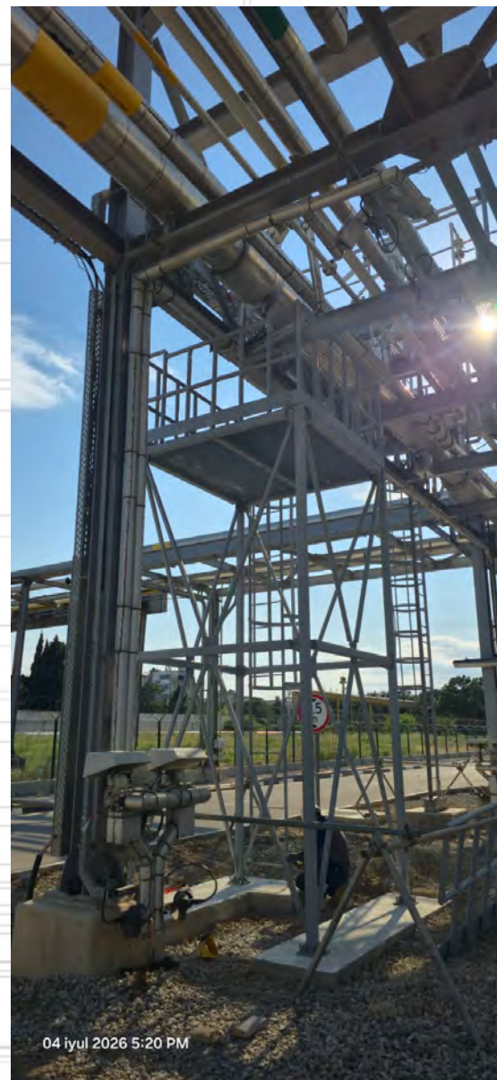
SOCAR Polymer: Installation of steam line meter platform (metal construction work)
