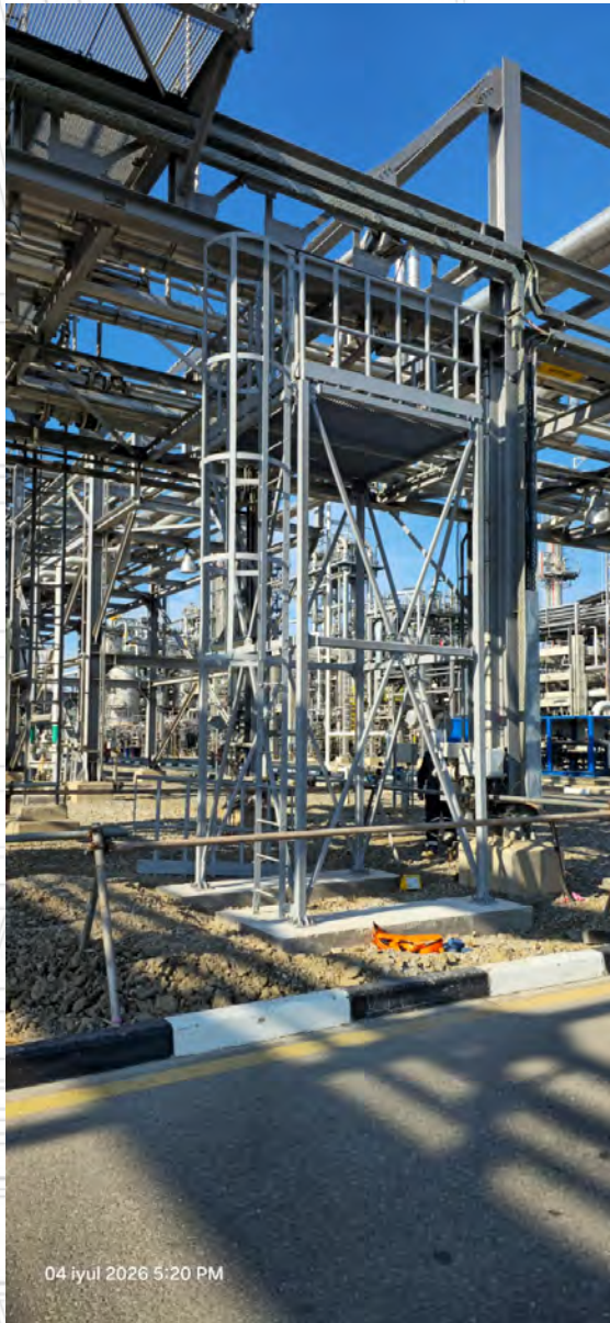
SOCAR Polymer: Installation of steam line meter platform (metal construction work)
