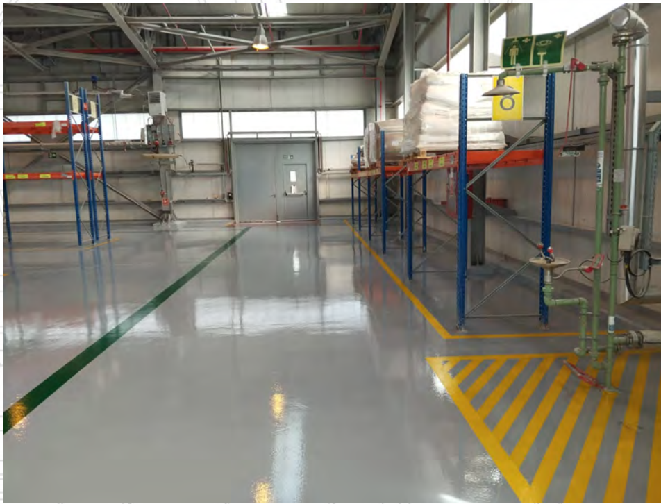
SOCAR Polymer: Epoxy coating of warehouse floor.
